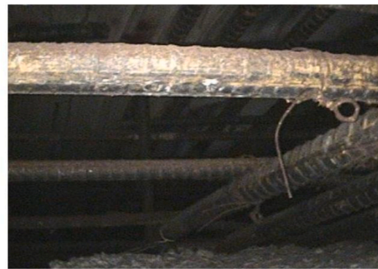
Fig. 19. Illustration of delamination location: (a) Diagram of delamination dimensions; (b) Image obtained from endoscopic imaging technique.
