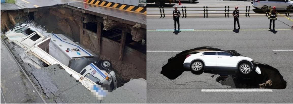
Fig. 1 Example of sinkhole formation in road structures leading to vehicle accidents (Source: Yonhap News)
